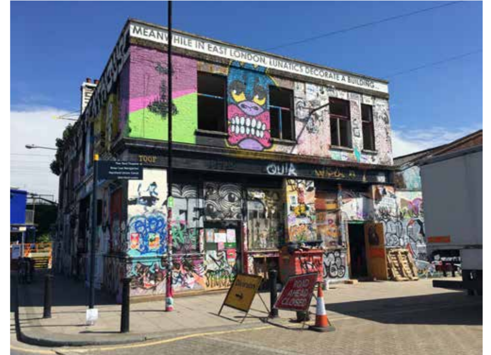
Existing view from White Post Lane
