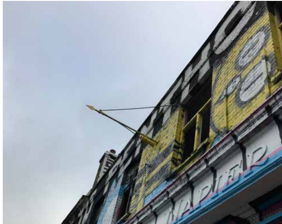
Existing brackets for hanging signs
